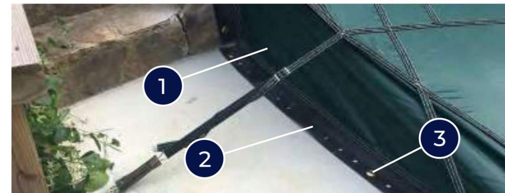
1. Triangular flap of mesh materials sewn to underside of cover.
